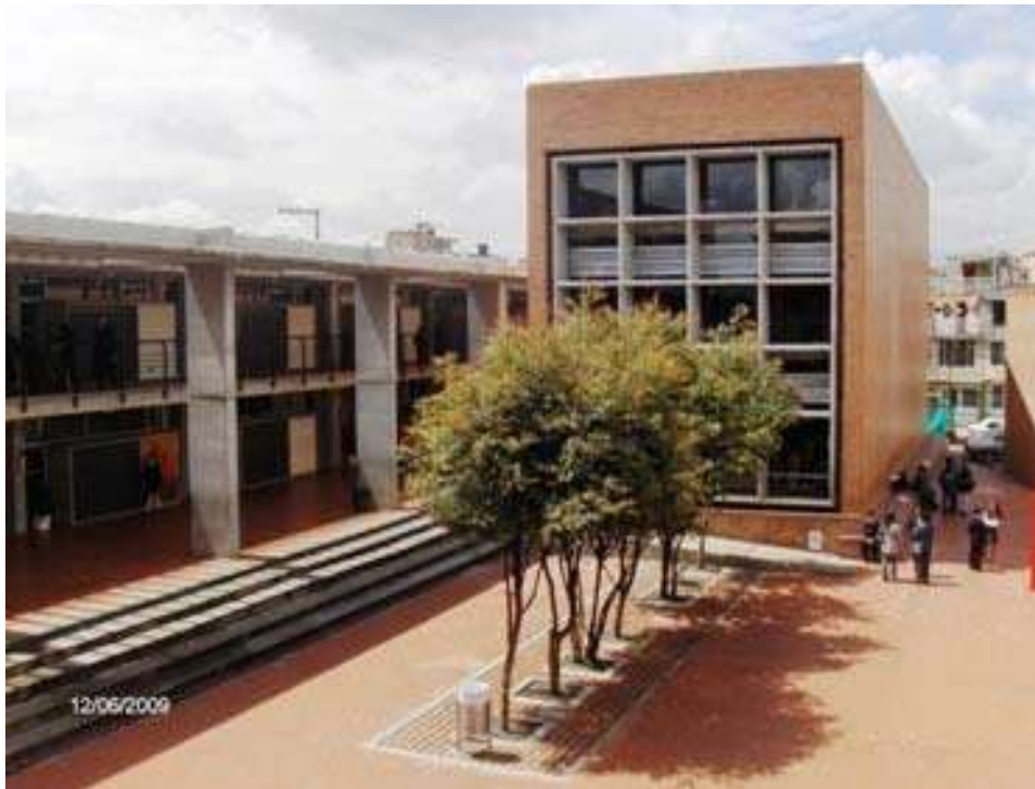
Figure 13: Public School Republica Dominicana. Architect Eduardo Samper by the Universidad Nacional de Colombia, Bogotá.
