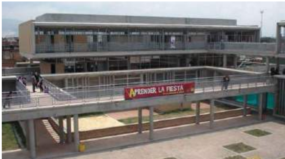
Figure 14: Public School Porfirio Barba Jacob. Architect: Leonardo Alvarez by the Universidad Nacional de Colombia, Bogotá
