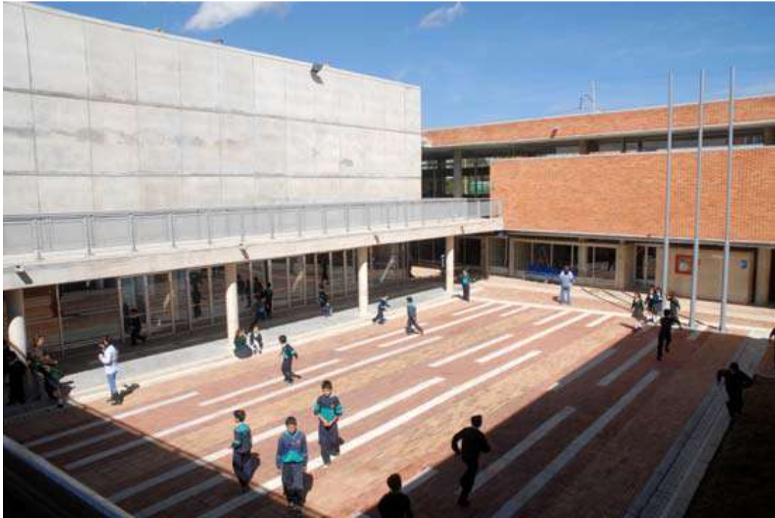
Figure 12: Public School Nicolas Buenaventura. Architect: Consorcio Arquitectura y Educacion Urbana. Leonardo Alvarez, Sergio Trujillo and Diego Suarez.
