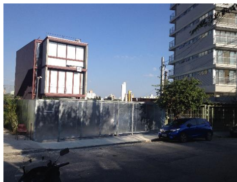
Window view in September 2015: all enclosed
