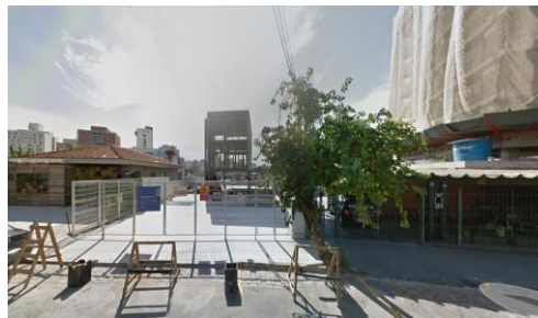
New constructions, November 2014
