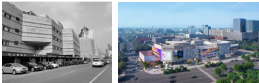
Before refurbishment, 2010s After refurbishment, 2023
