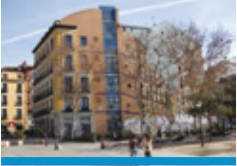
7. APR: Four Squares – new and old buildings at de los Carros Square
