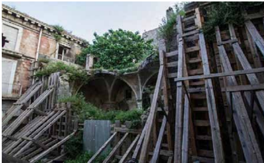
Figure 8. The state of the Church of San Paolo 14 years after the collapse
