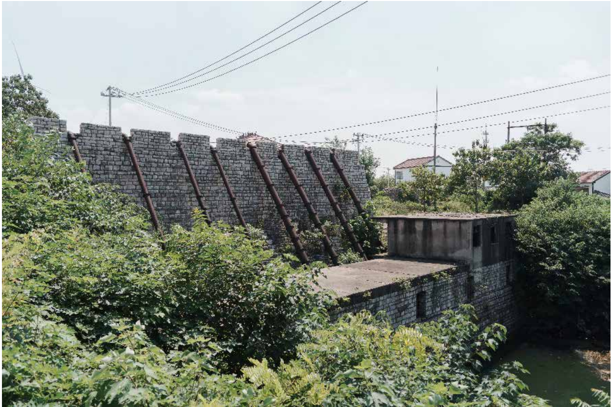
Figure 6 Desalination plant still in use.
