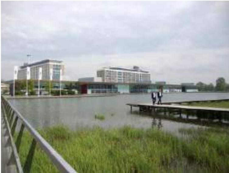
Figure 5. High Tech Campus Eindhoven: The Strip and walking route around the pond
