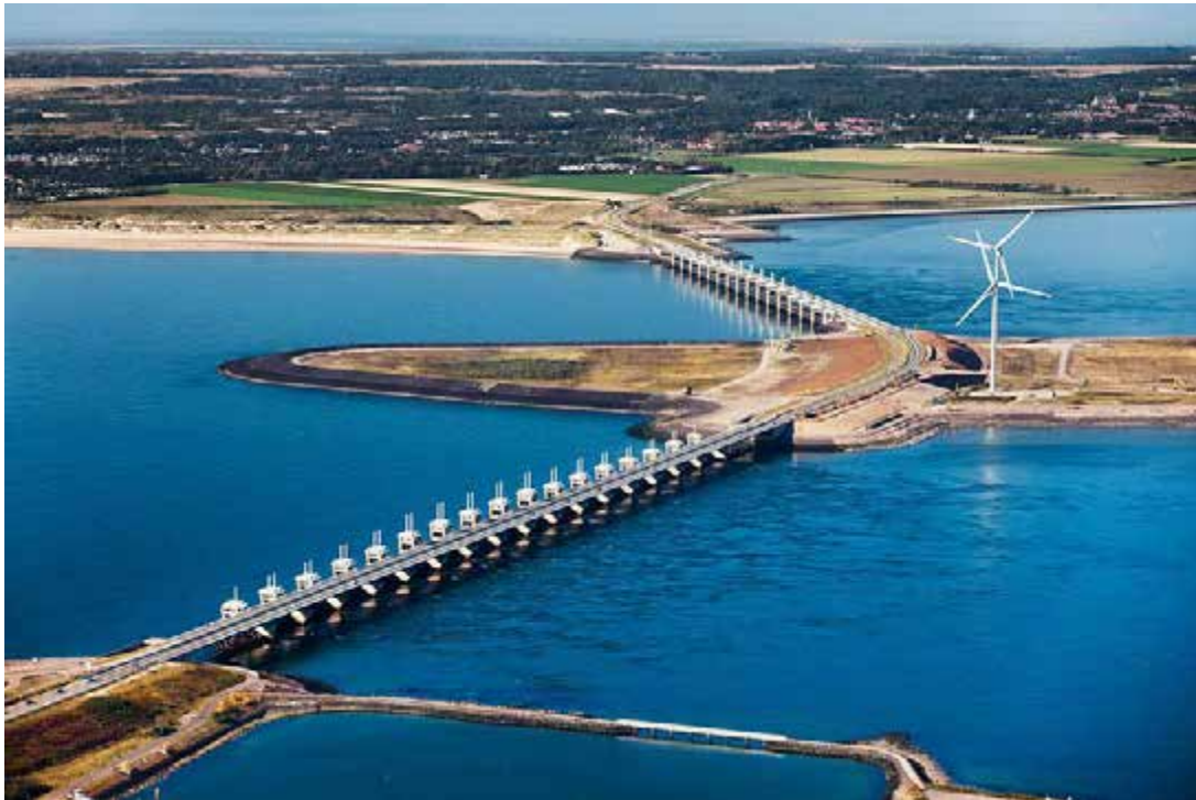
Fig. 4: Aerial photo of Oosterscheldekering flood barrier by Frans Lemmens
