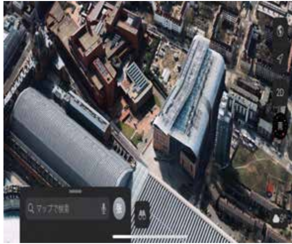
Figure 10: Aerial view of the Francis Crick Institute (Source: Apple 3D Maps).
