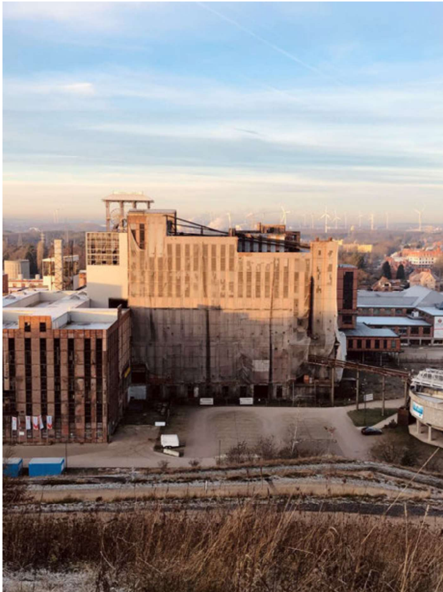
Figure 1. Part of mine site with huge coal washing plants
