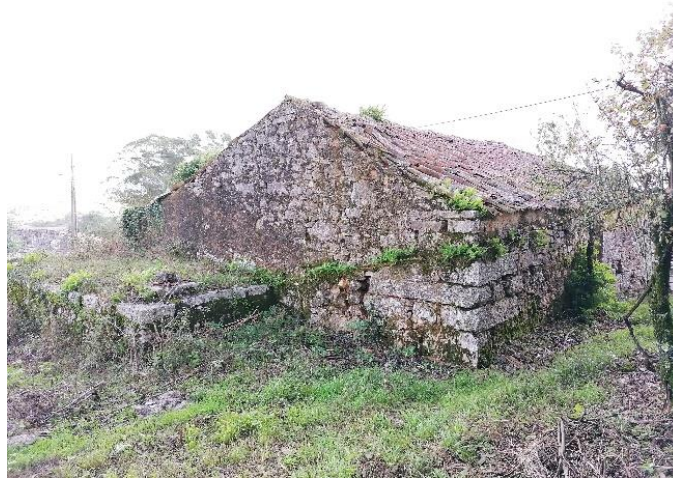
Figure 10. Tanks outside of the building, visible the channel conducting the water from the roof
