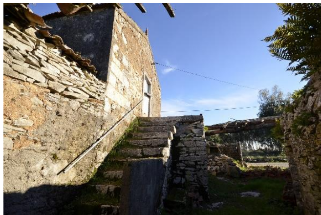
Figure 7. Cisterns for rainwater storage under the stairs in Chanca
