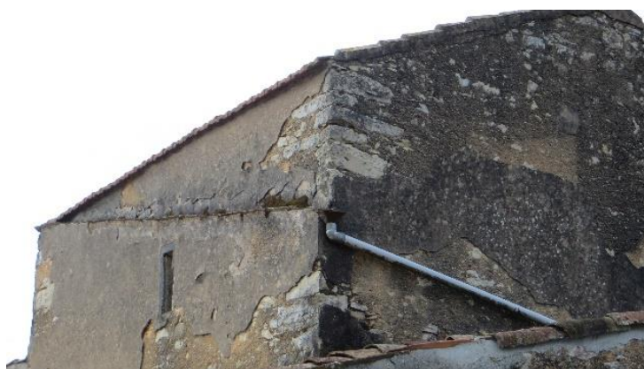
Figure 8. System of channel and pipes conducting the water from the roof
