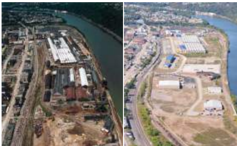
Figure 3.1. Past and current uses of McKeesport Brownfield redevelopment site. Available at http://www.ridc.org/files/a_files/Case%20Study%20-%20McKeesport%20-%20red.pdf
