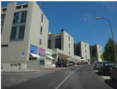
3. Active façades, Sanchinarro
