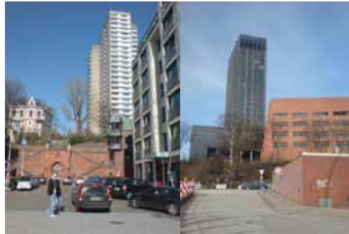
18. Historical parts of the collective Wasserschutzmauer
