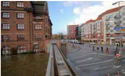
16. At strategic spots, Hamburg has 'flood gates' as part of a collective protection system
