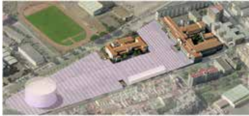
4. University of La Laguna – Central Campus with the new Resource Centre for Learning and Research
