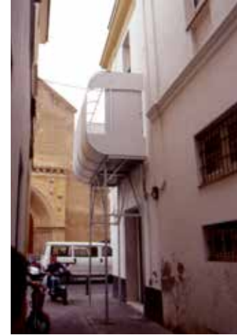
2. Scaffolding project built in the historic district of Seville.
