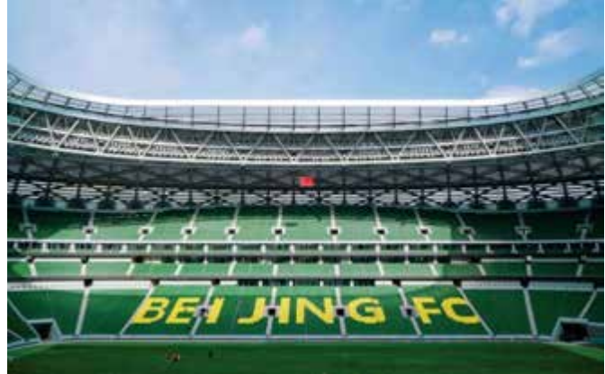
Figure 12: Inside New Workers Stadium
