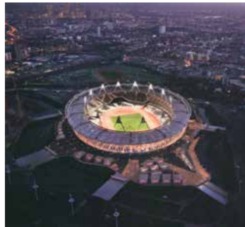
Figure 21: London Olympic Stadium
