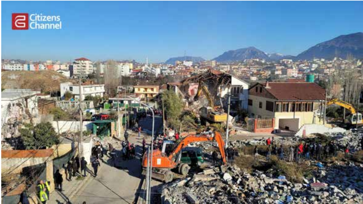
Figure 5: The demolition operation of 5 Maji neighborhood. Source: Citizens.al, Facebook 09.02.2022
