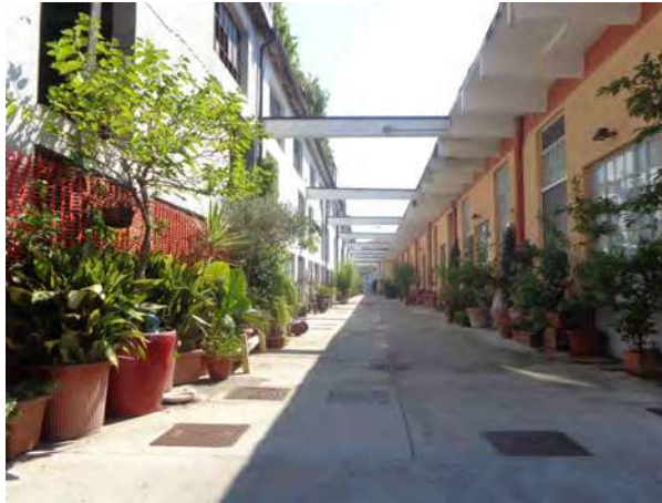
Figure 3. A street inside Tucidue56 area, result of the operation of subtraction and cut of a former warehouse.
