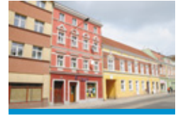
13. Renovated row of tenement houses in Psie Pole
