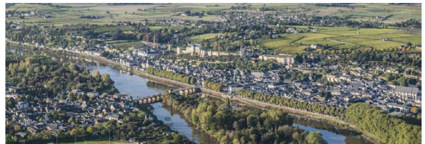
3. The monumental site seen in its contemporary urban context.
