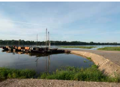
16. The restoration of the Possonière Port, with its discrete quay extension, has been adapted to the Loire's low-water periods.
