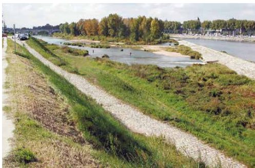
5. The duit Saint-Charles, port of Orléans: the maintenance problems posed by channeling work on the Loire (lowest water level).
