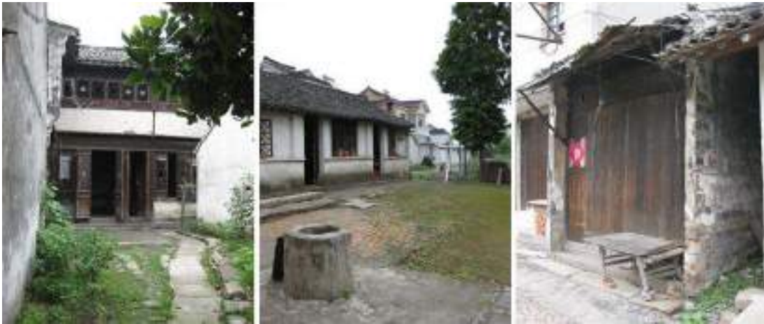
Figure 7. Dilapidated and abandoned houses in the Jinshi village.
