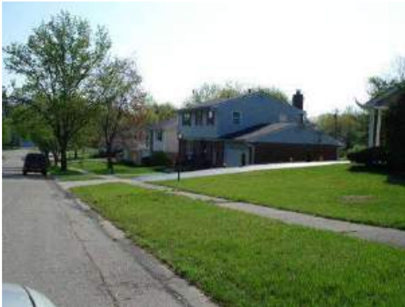
Figure 12. Larger single family detached homes along a Forest Park street
