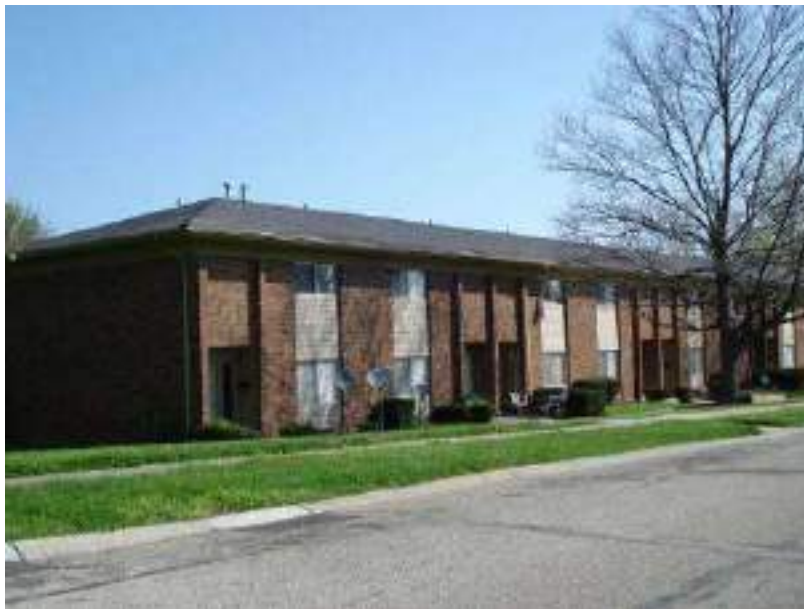
Figure 37. Forest Park Apartments, low-rise complex containing voucher residents
