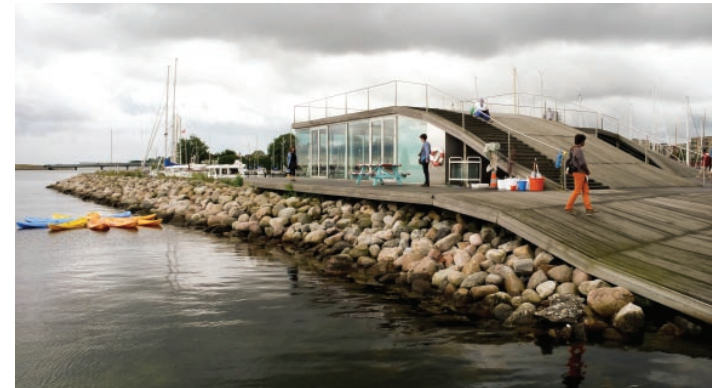
13. Maritime Youth House in Sundby Harbour.
