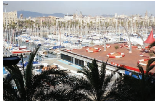
5. Hangar's roof serving as a public space.
