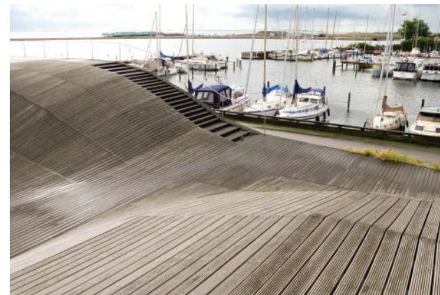
15. Maritime Youth House in Sundby Harbour.
