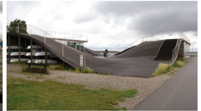
14. Maritime Youth House in Sundby Harbour.
