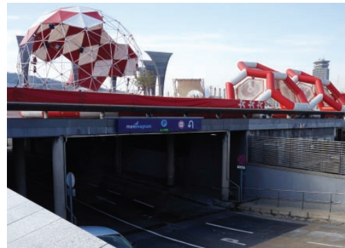
4. Bridge over the street connecting hangar's roof with public space. Photo by Katarzyna Rembarz
