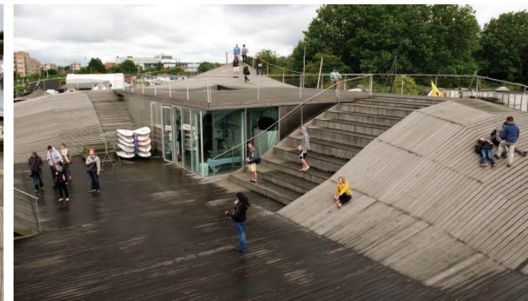
16. Maritime Youth House in Sundby Harbour -people enjoying wooden deck.
