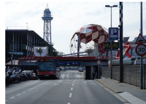
3. Bridge over the street connecting hangar's roof with public space.
