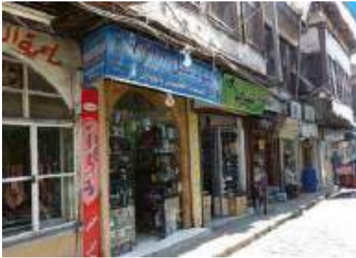
Photo 4: Boxes hiding Arches
