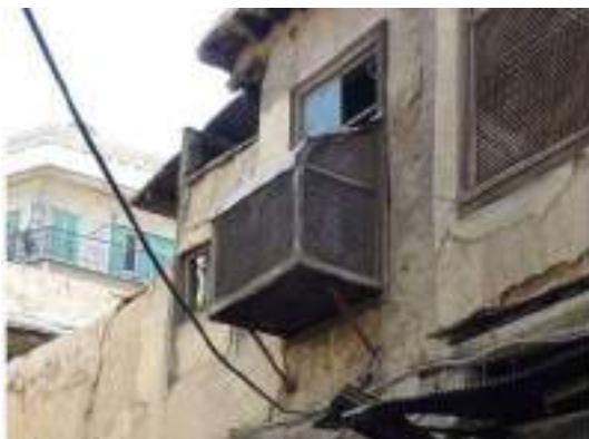
Photo 6: Electricity Cables on Hus
