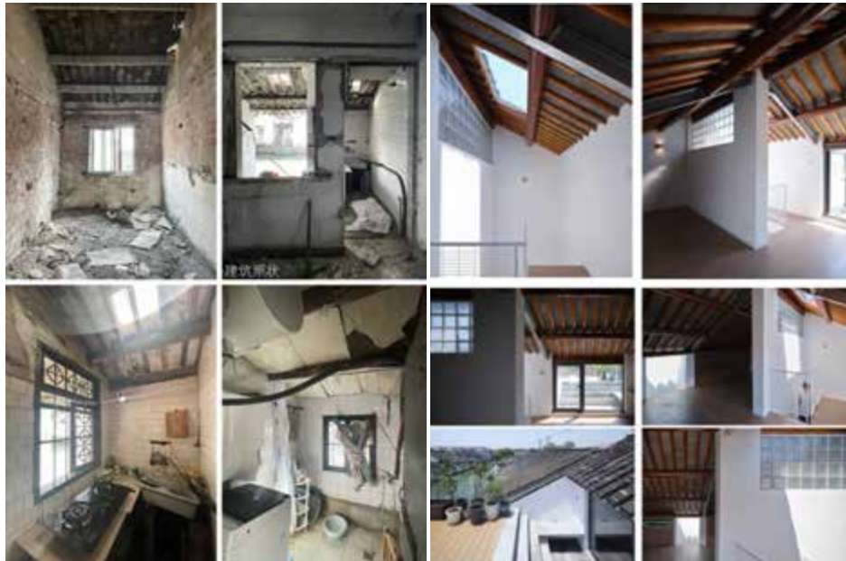
Fig 14-15. An example of the renovation of a traditional residential building located on Shantang Street in the ancient city of Suzhou 2024 Picture source: DEKONG STUDIO
