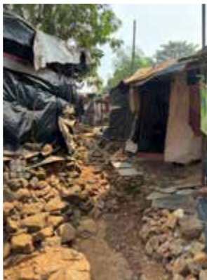
Fig 6. Tenements on site (Photo by author)
