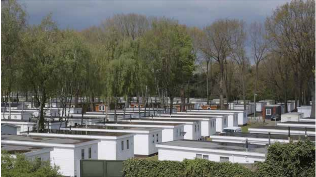
Fig. 01 Typical mobile home park to accommodate migrant workers, North Brabant region, Netherlands. Photo by the author.
