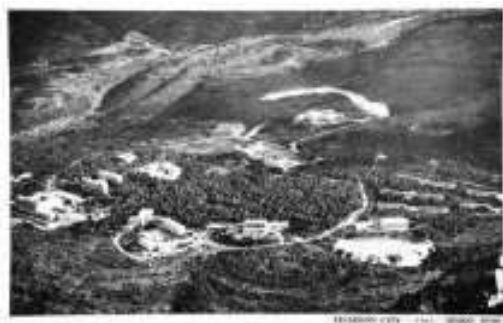
Figure 1: Aerial photograph of Technion campus, circa 1962
