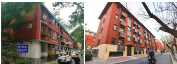
Figure 2. Before and after regeneration of No. 17 Guangminglou Residence (Source: https://baijiahao.baidu.com/s?id=1751087758495236894&wfr=spider&for=pc )
