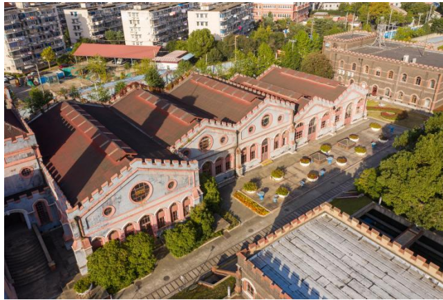
Figure 5. Aerial View of the Buildings at Yangshupu Water Plant
