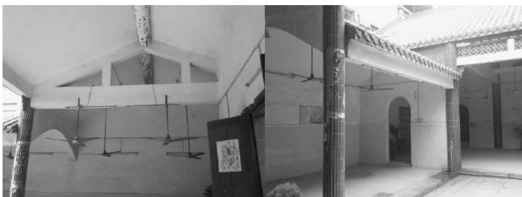
Figure 9 –Cement beam Figure | 10 – cement column stuck with tile
