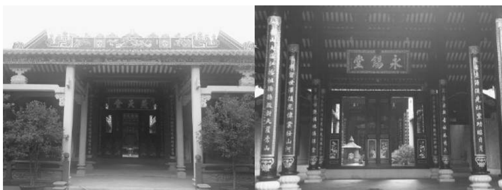
Figure 11 –Cement beam Figure | 12 –Wood structure
