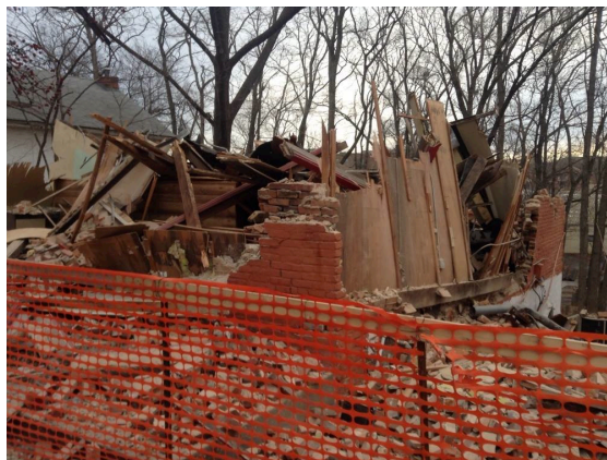
Figure 4. Cottage demolished on December 25-26, 2014. [Photo by Tom Gilseman]
