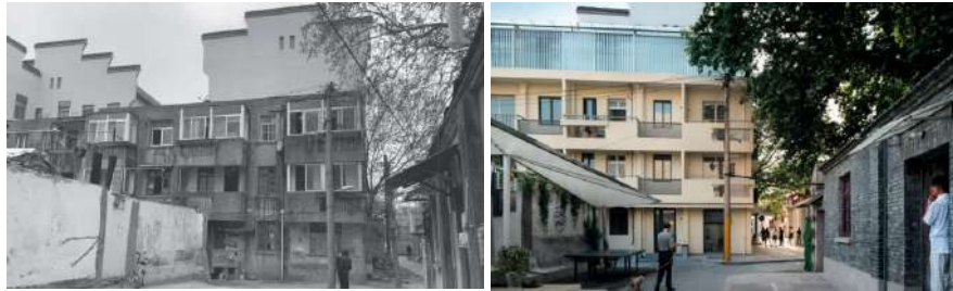
Fig. 7. Pre- and post-renovation relocation housing
