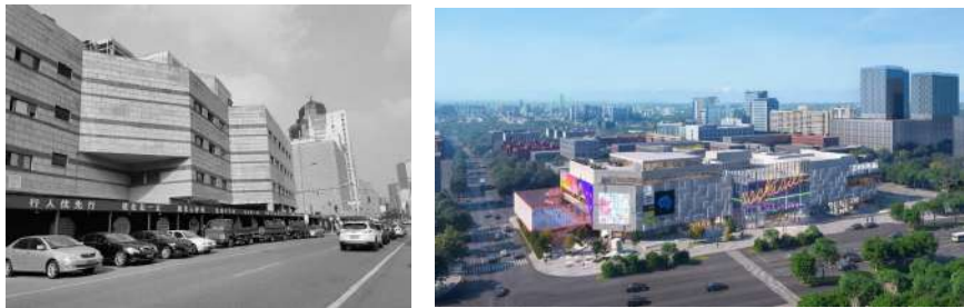
Before refurbishment, 2010s After refurbishment, 2023 Fig. 8 Real scenes of BOX Chaowai, Beijing
