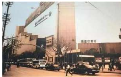
Before Refurbishment, 1990s
