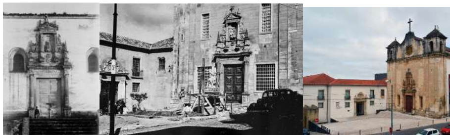
Figure 3 - Portal of Santa Ana in its original location (early 20th century) [AMNMC, Photographs folder]. Figure 4 - Its reuse in the S. Salvador Church (c.1930) [AMNMC, Photographs folder]. Figure 5 – St. Salvador Church today
