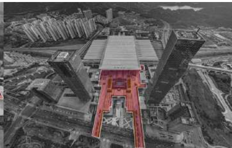
Fig 4. Aerial view of the Over-rail Plane of Shenzhen North Station Source: Drawn by Author
