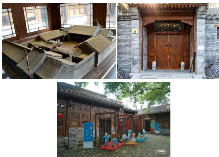
Figure.1 No.23 House of Shijia Hutong, originally used for residential purpose, now converted into Shijia Hutong Museum
