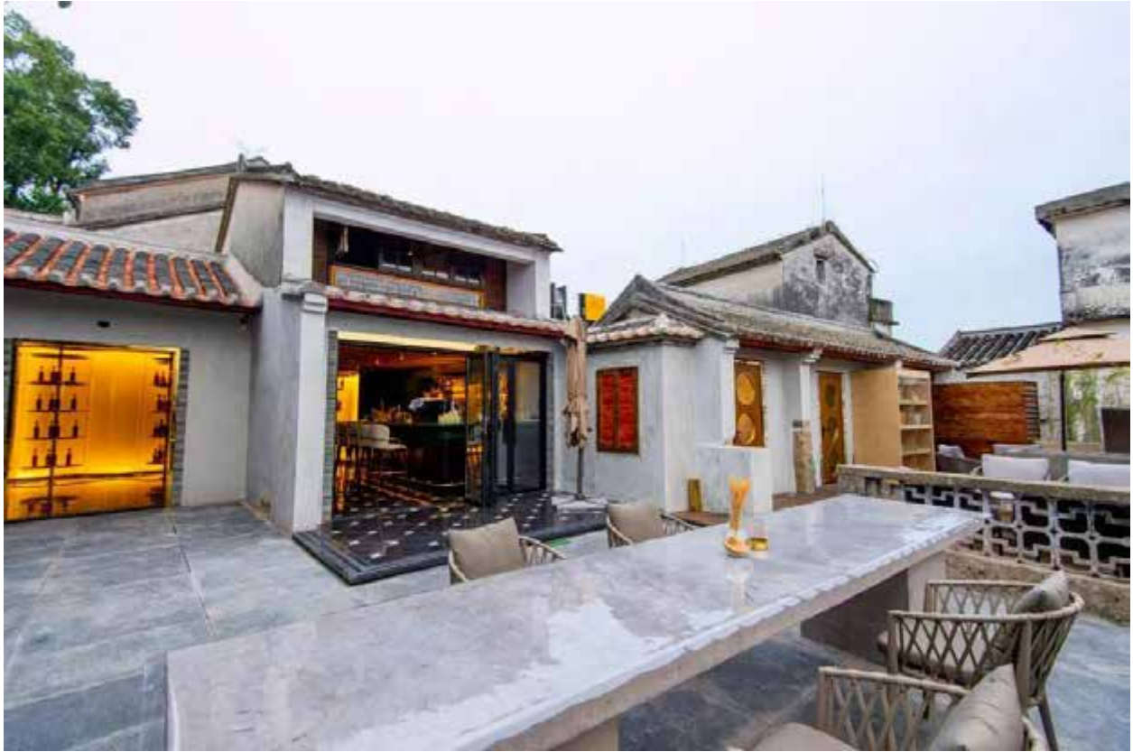
“original appearance protection” + “function regeneration” of Shenzhen Dapeng Fortress source from sznews.com
