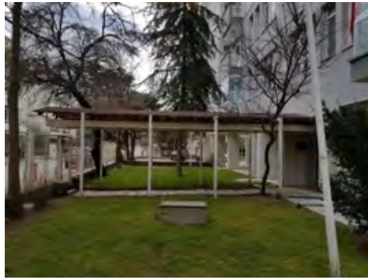
Figure 24- Building entrance, relation with the street
