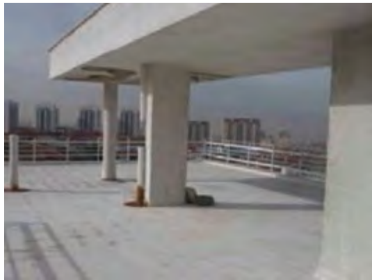
Figure 28- Roof level (Source: Sudaş, 2010)
