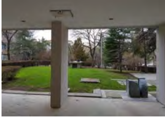
Figure 25-The buildings are lifted from the ground with pilotis.
