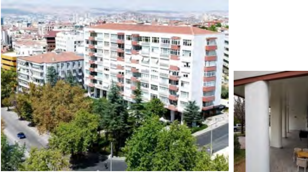
Figure 6- The Hayat Building lifted from the ground on pilotis (Source: Social media page for the building)
