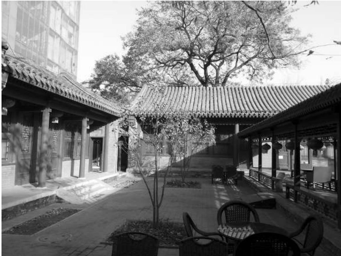
Figure 5. Courtyard of a Siheyuan filled with various small extensions that meet the growing needs of living space for more dwellers. (photo Marlène Leroux)
