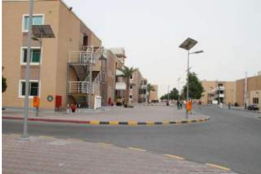
Figure 2: Overall view of some dormitory buildings
