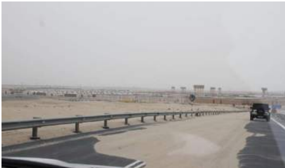
Figure 1: Al-Raha Worker City main approach road
