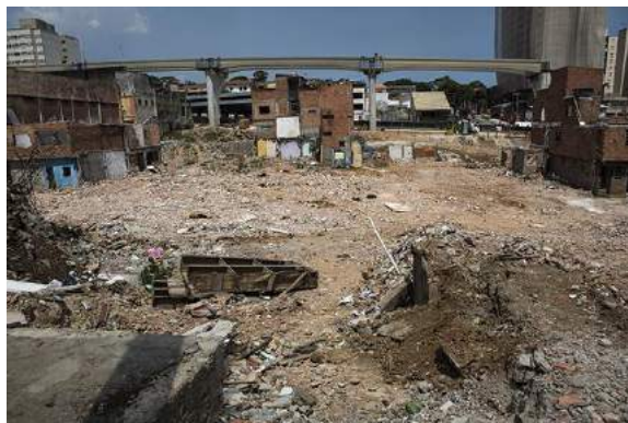
Figure 1 – Favela removed for mobility works in São Paulo. Source: https://www.vice.com/pt_br/article/esses-sao-os-resistentes-das-desapropriacoes-da-favela-buraco-quente
