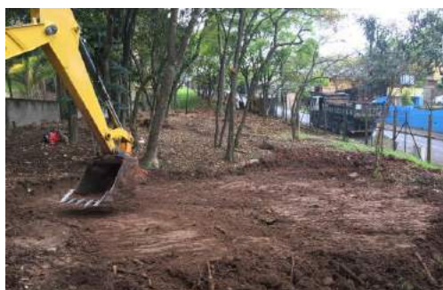
Figure 6 - Construction of the Park in Jardim Jaqueline Source: FAU Social collection
