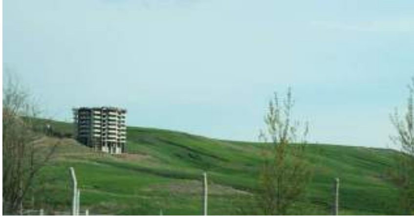
Figure 10. TOKİ Turkuaz Konutları, West Corridor, 2010, Personal Archive.
