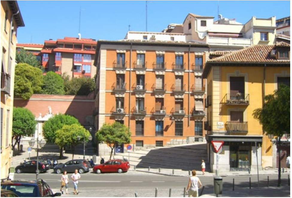
Figure 2-9 Urban improvements in residential and commercial areas. Source: Teresa Franchini.
