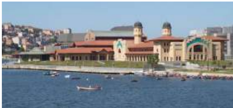
Figure 3. Sutluce Slaughterhouse, after reconstruction (Source: Z. Günay)
