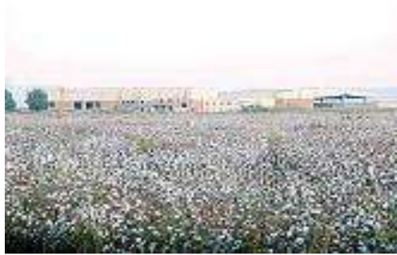
Figure 15. The Existing Waste Facility in Menemen between Agricultural Lands with Quality (YA, 30.12.2011)
