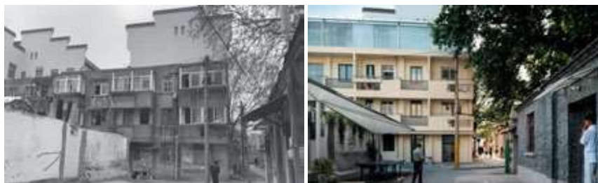
Fig. 7. Pre- and post-renovation relocation housing
