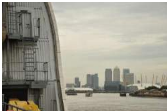
Figure 4. Thames Barrier and Canary Wharf, Source: Author, August 2011
