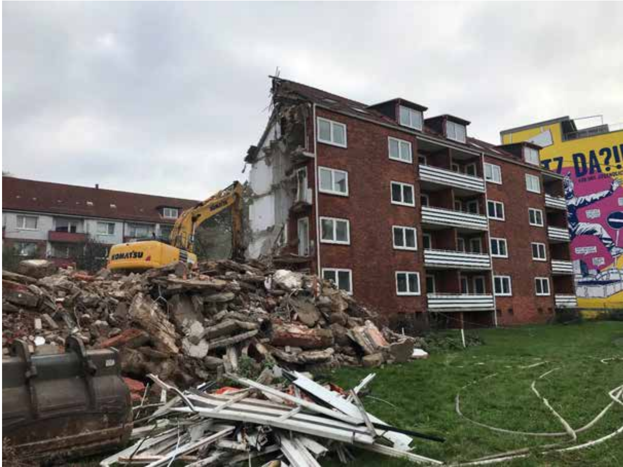
Figure 1: Demolition of a multi-family building from the 1950s and 1960s, Billhorner Röhrendamm (Hamburg)
